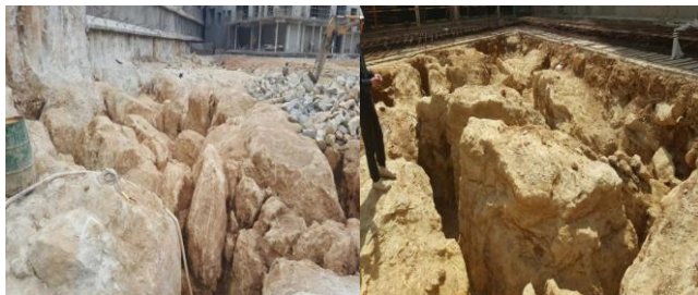
Fig.3. Karst conditions exposed after foundation pit excavation to formation level
